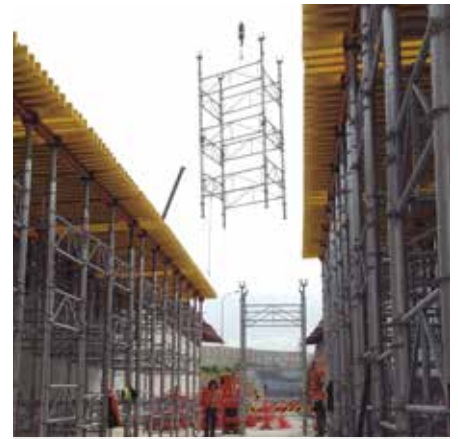
ALUPROP tower lifting
