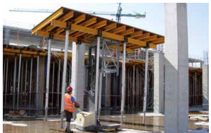
VR Table pre-assembled slab formwork with ALUPROP prop
