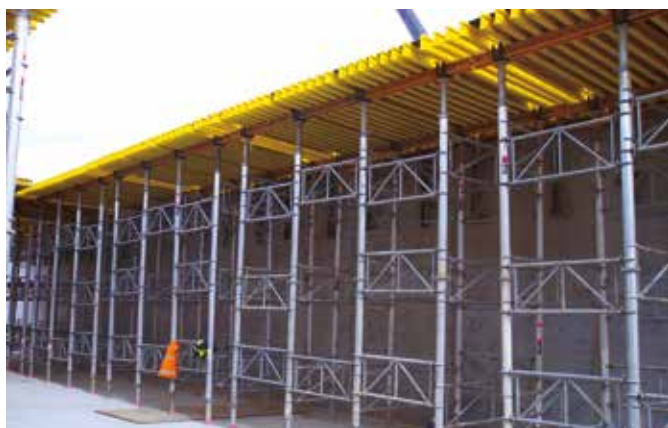
VR Table pre-assembled slab formwork with ALUPROP towers
