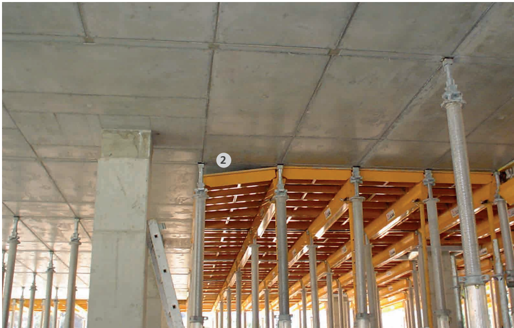
1 Efficient performance in terms of assembly due to the system's lightness. 2 Stripping with the drophead.
