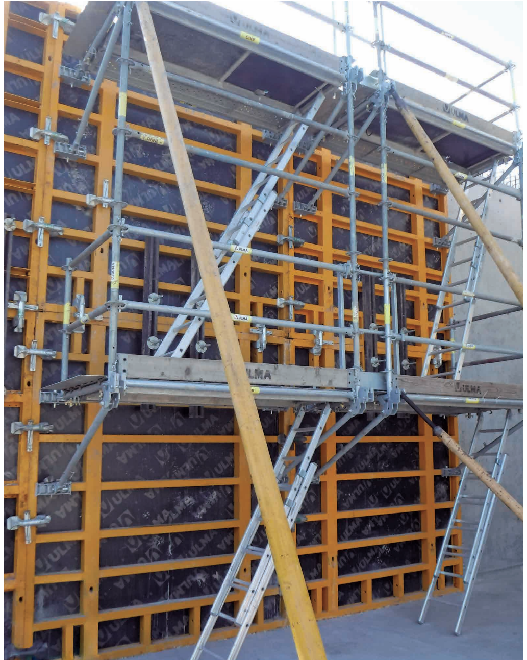
2 Platforms made of non-slip perforated sheet.
