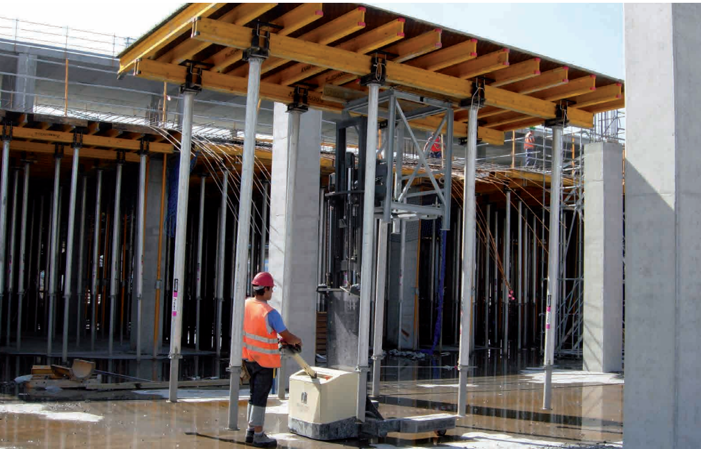
1 Incorporated handrails on perimeter tables for the entire process.
