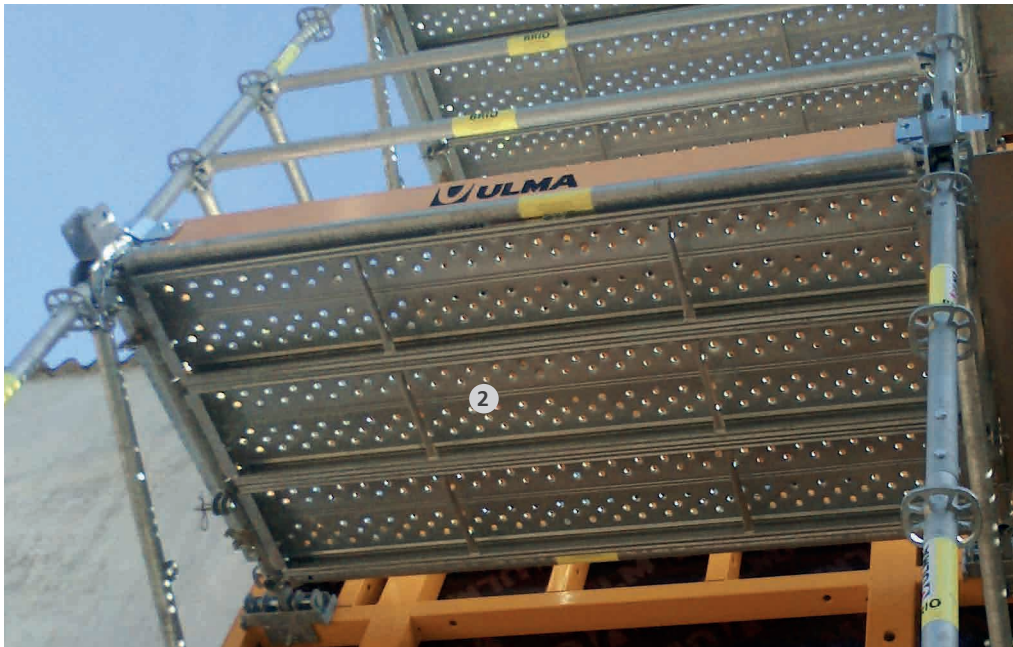
1 Joint between panels and SBU platform using heads (pictured) or walers.
