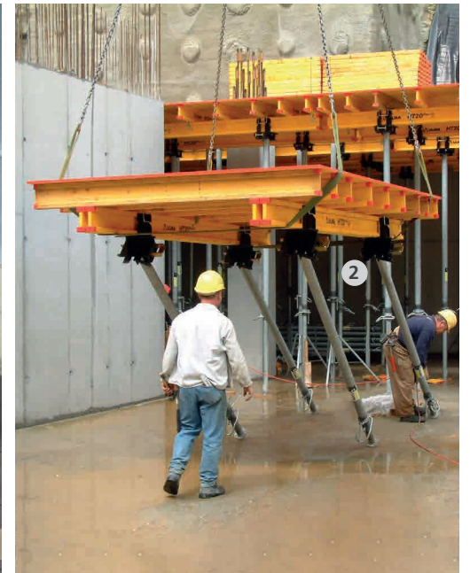
2 Swivel head for folding the props and thus easily going around obstacles or parapets when moving the tables.
